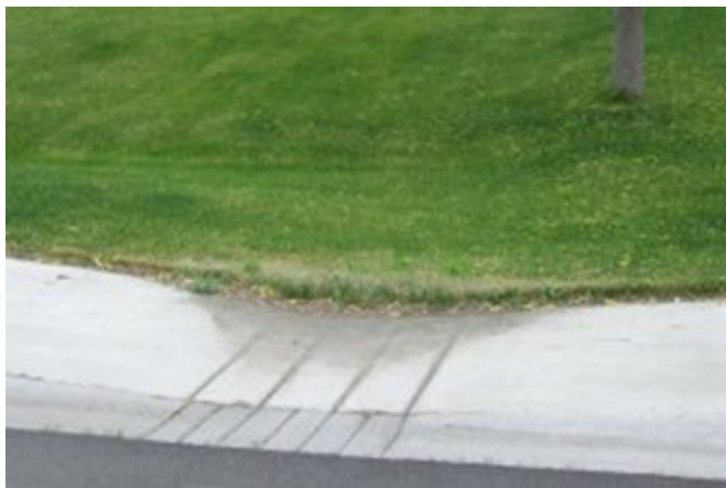
Figure 2 - Front yard bioswales illustrating sloped sidewalks, curb openings, and graded lawn depressions
