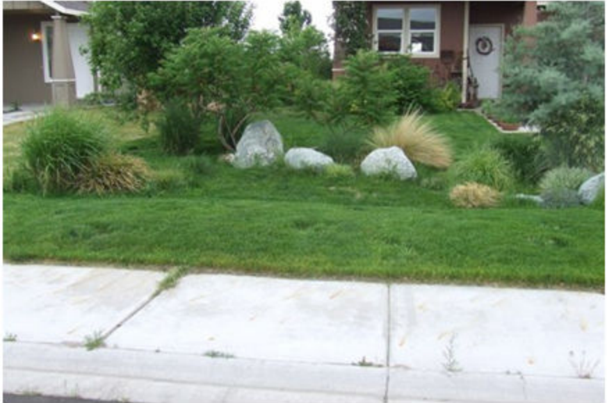
Figure 4 - Front yard bioswale incorporated into the landscape
