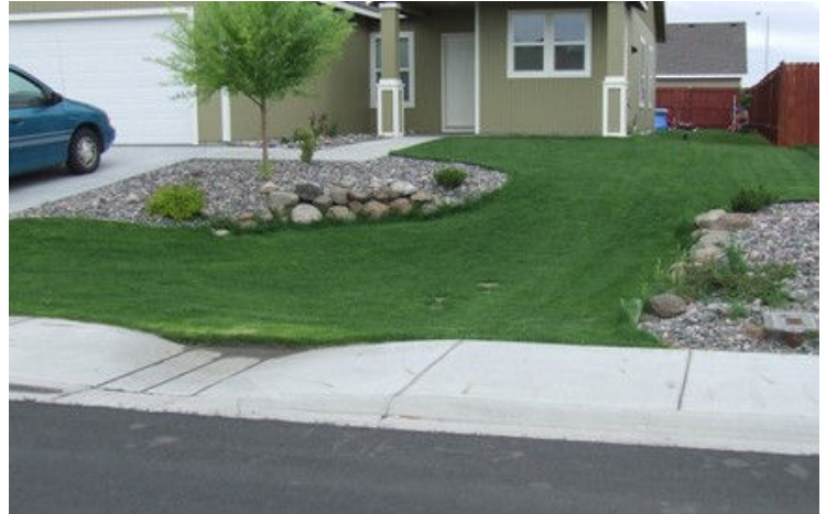
Figure 1: Front yard bioswales, sloped sidewalks, curb openings and depressions.
