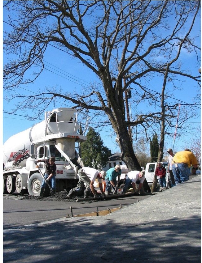
Installation of the pervious concrete.
