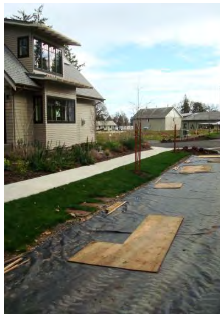
Figure 6: Geotec Fabric on the permeable pavement for protection during home construction.
