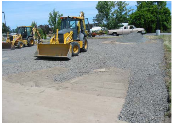
Figures 3 & 4: Showing the construction of the sub-base for the grassy pavers
