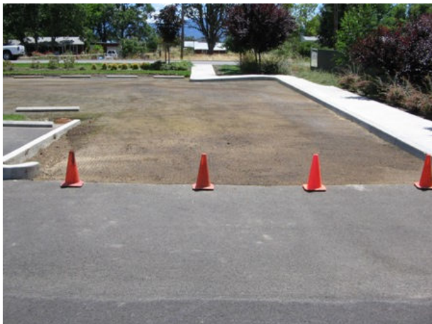
Figures 3 & 4: Showing the construction of the sub-base for the grassy pavers
