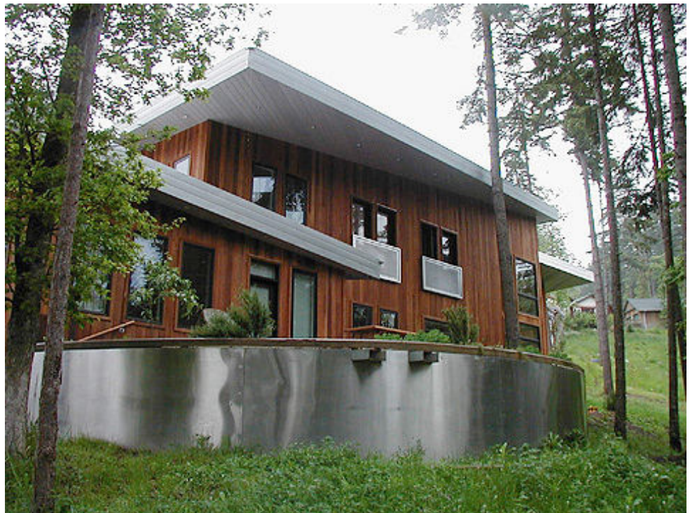
The metal clad, cement cistern can store 8000 gallons.
