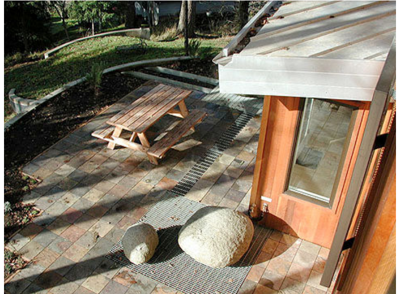
Rooftop runoff is directed onto boulders and grates where it is then filtered before running into a cistern. Photo by Eimar Boesjes.
